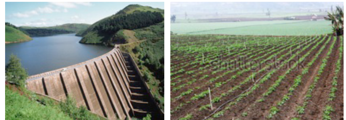
Water dam and reservoir
