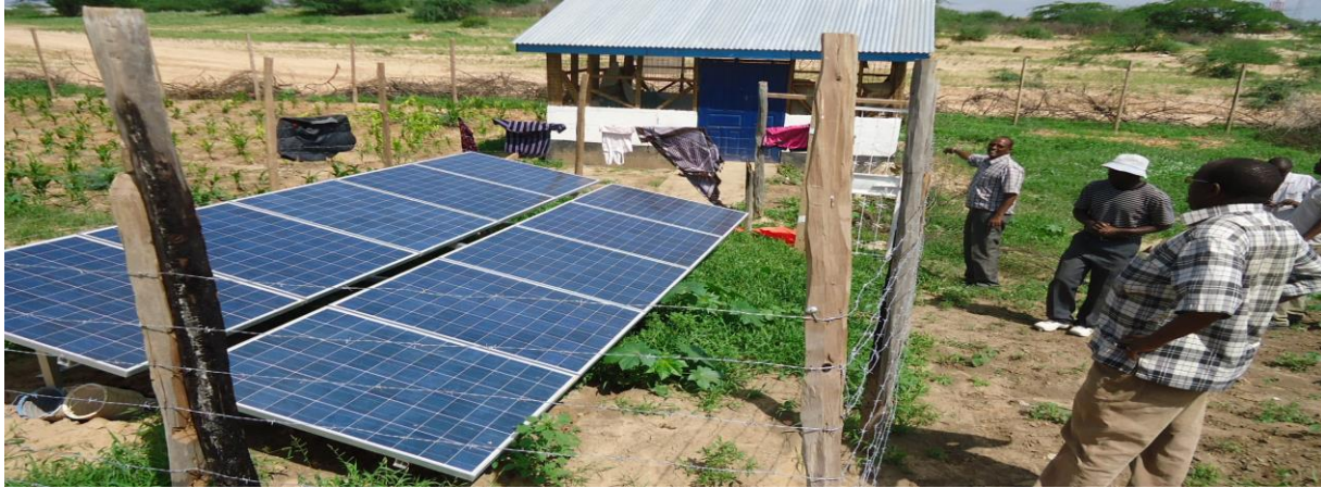
Figure 9: Solar panels in Ashabito Water Pan
