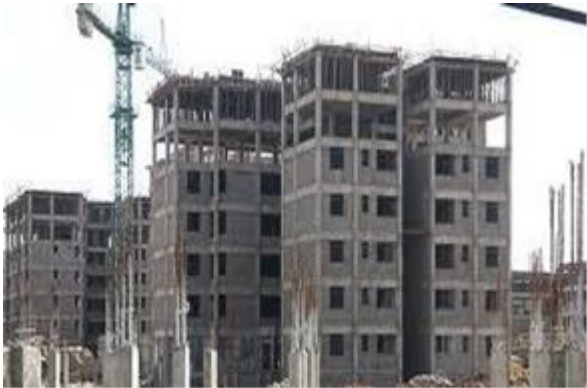
Nation Apartments under construction in Nairobi. Nation Media File
