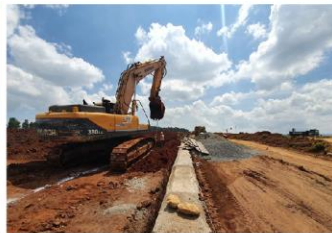
Phase II construction ongoing
