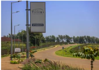
Completed Phase I infrastructure
