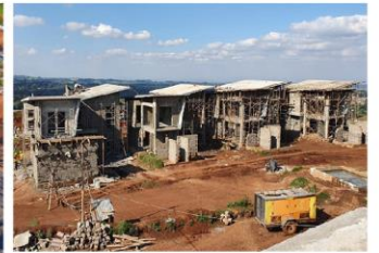
Ongoing construction of Tilisi Views
